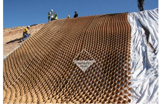
FIGURE 1 - INSTALLATION OF NEOLOY GEOCELLS
