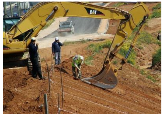
FIGURE 4. CLEAR AND SHAPE SLOPE
