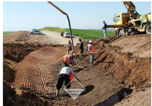
FIGURE 21. POURING CONCRETE INFILL OF TRENCH
