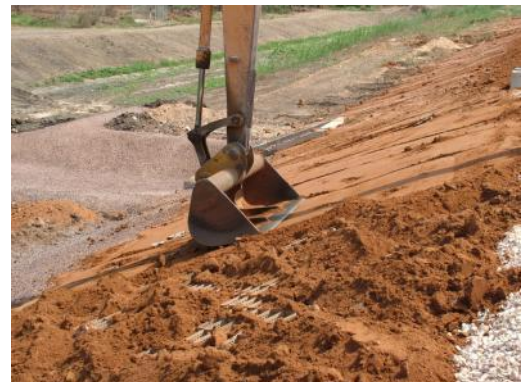
FIGURE 19. BLADE COMPACTION
