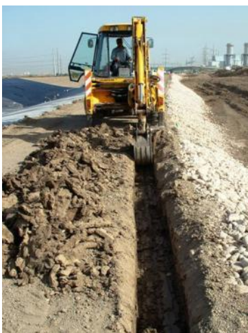
FIGURE 6. EXCAVATING TRENCH AT TOP OF CREST
