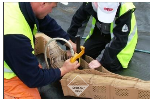
FIGURE 13. FASTENING END TO END
