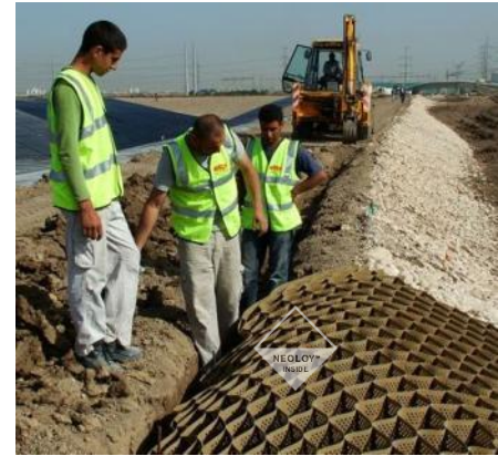
FIGURE 15. PLACING SECTION ON ANCHORS AT CREST
