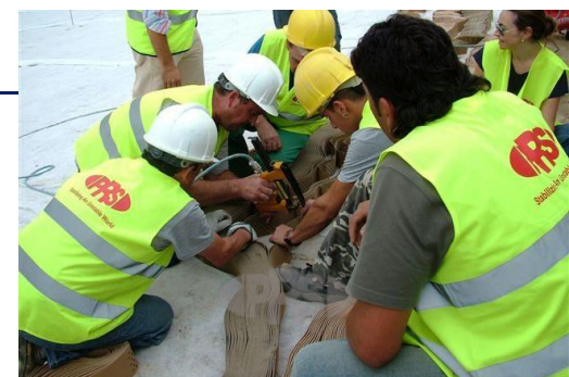
FIGURE 14. FASTENING SECTIONS FACE TO FACE
