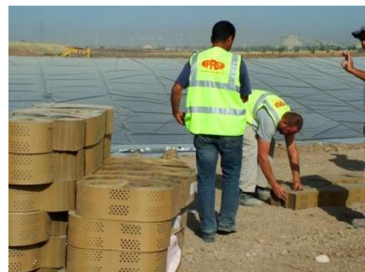
FIGURE 3. OFF-LOADING SECTIONS ON-SITE
