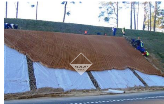
FIGURE 17. EXPANDING SECTIONS DOWNSLOPE
