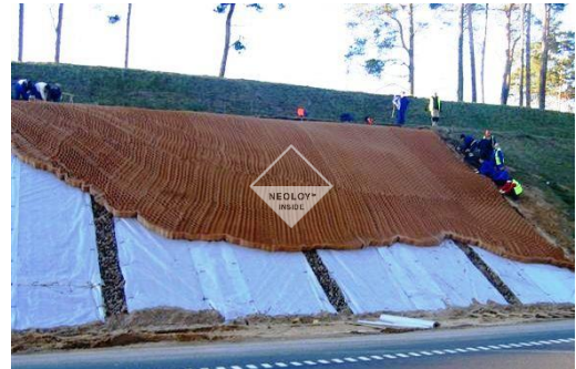
FIGURE 24. DOWNSLOPE DRAINAGE SPILLWAYS
