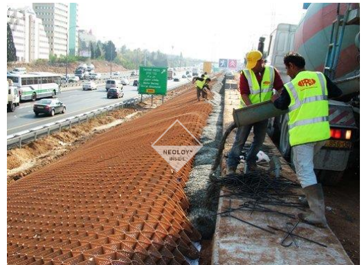
FIGURE 20. CONCRETE INFILL OF CREST TRENCH
