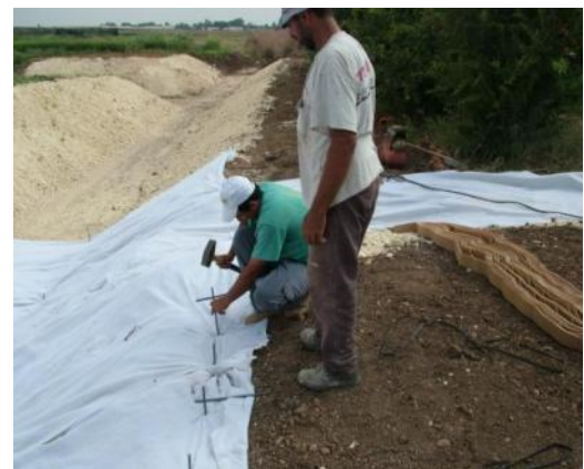
FIGURE 8. ANCHORING STAKES
