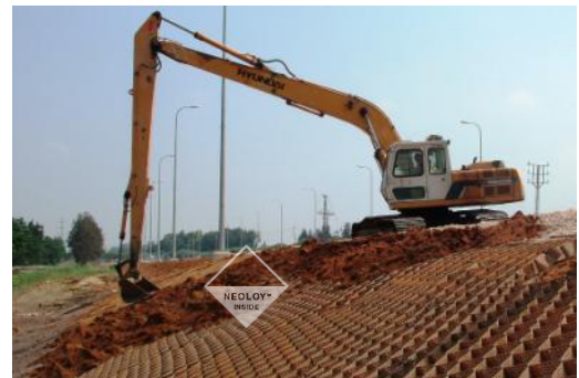
FIGURE 18. SOIL INFILL DOWNSLOPE BY EXCAVATOR
