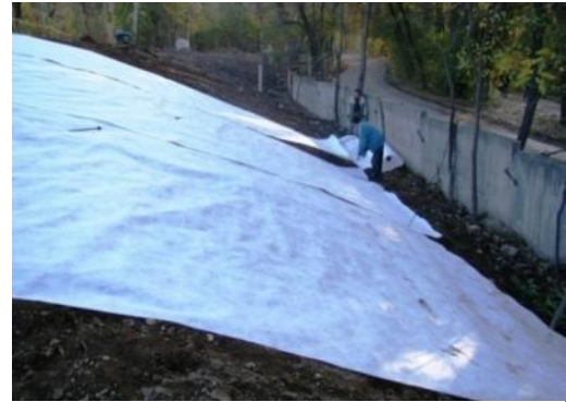
FIGURE 7. LAYOUT TEXTILE
