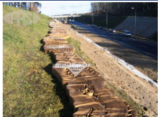
FIGURE 11. LAYOUT SECTIONS ALONG CREST SLOPE
