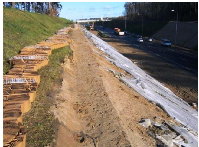
FIGURE 5. TRENCH ALONG SLOPE CREST
