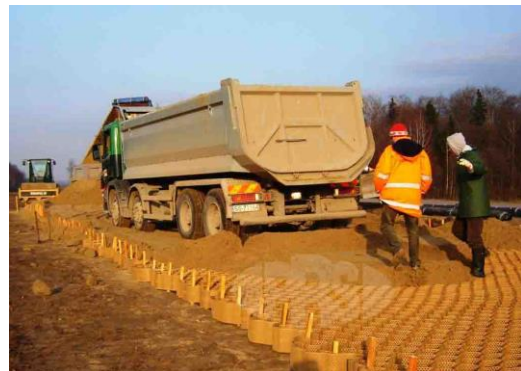
FIGURE 16. INFILL PLACEMENT
