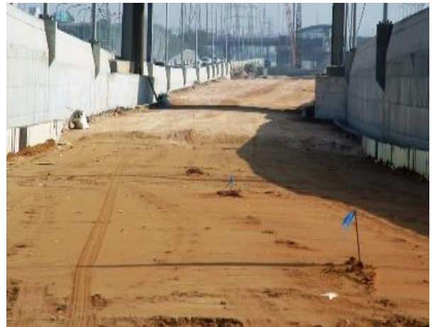
FIGURE 3. PREPARE SUBGRADE LAYER
