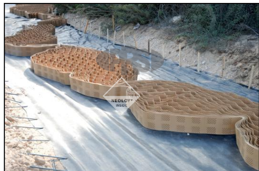
FIGURE 7. LAYOUT SECTIONS ALONG ROAD LENGTH
