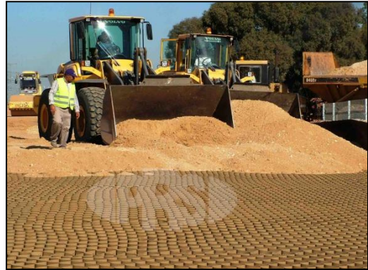
FIGURE 15. SPREADING INFILL
