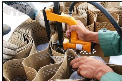
FIGURE 10. FASTENING SECTIONS FACE TO FACE
