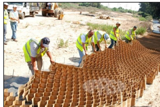
FIGURE 12. EXPANDING SECTIONS OVER ANCHORS
