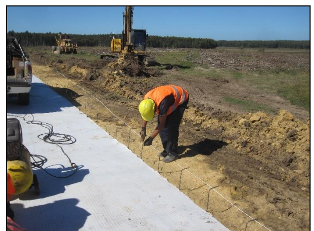
FIGURE 5. INSERTING STAKES/ANCHORS ALONG ROUTE
