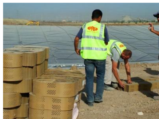
FIGURE 2. OFF-LOADING SECTIONS ON-SITE
