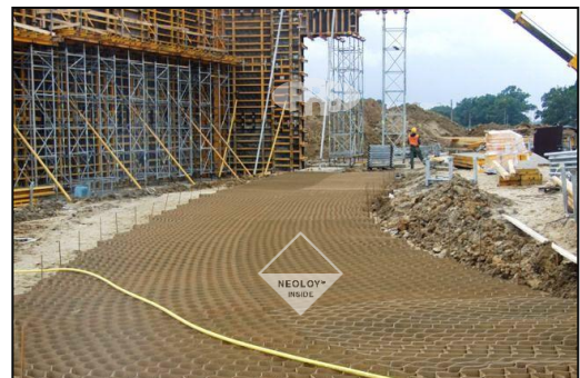
FIGURE 14. INSTALLING SECTIONS ON CURVES
