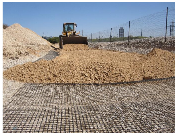
FIGURE 4. LAYOUT GEOTEXTILE
