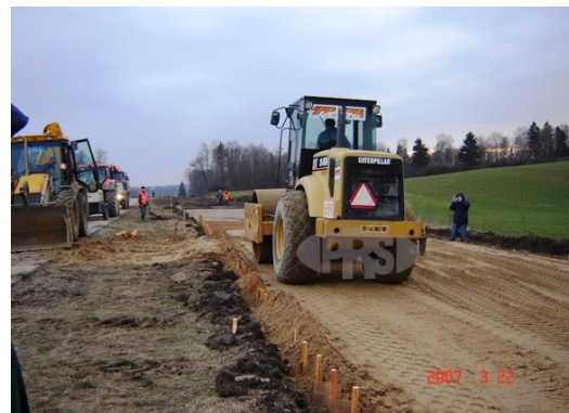
FIGURE 18. COMPACTION
