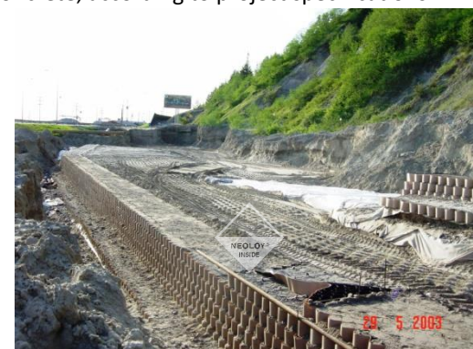
FIGURE 19. BACKFILL OF BACK SLOPE
