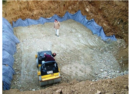
FIGURE 7. PREPARATION OF BASE LEVELING PAD
