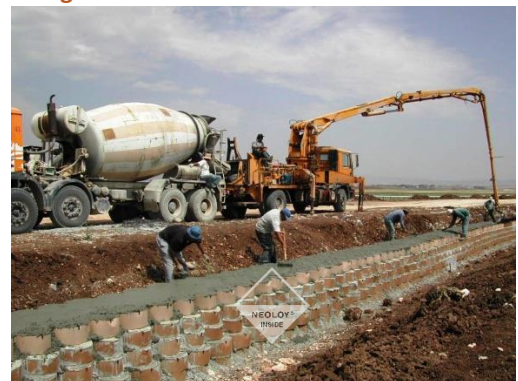
FIGURE 18. INFILL PLACEMENT
