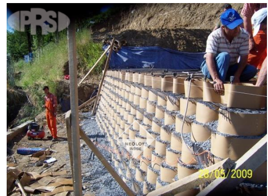
FIGURE 15. POSITIONING GEOGRID REINFORCEMENT ALONG LENGTH OF WALL
