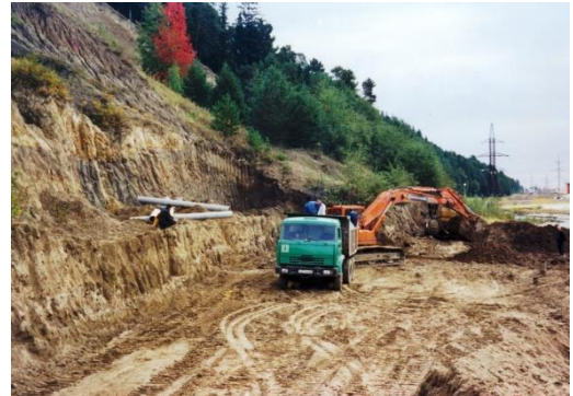
FIGURE 4. PREPARE SUBGRADE LAYER
