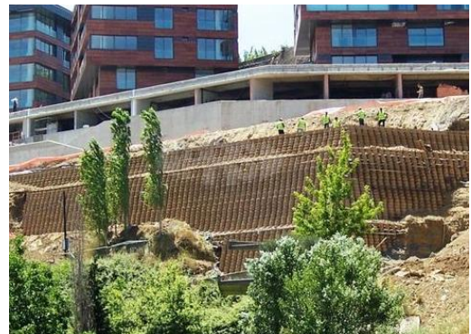
FIGURE 1 - INSTALLATION OF NEOLOY
