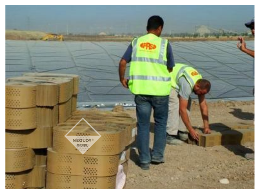
FIGURE 3. OFF-LOADING SECTIONS ON-SITE
