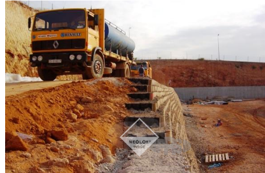
FIGURE 20. WATERING INFILL FOR COMPACTION
