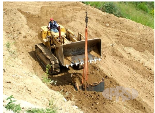
FIGURE 5. EXCAVATING FOUNDATION SOIL
