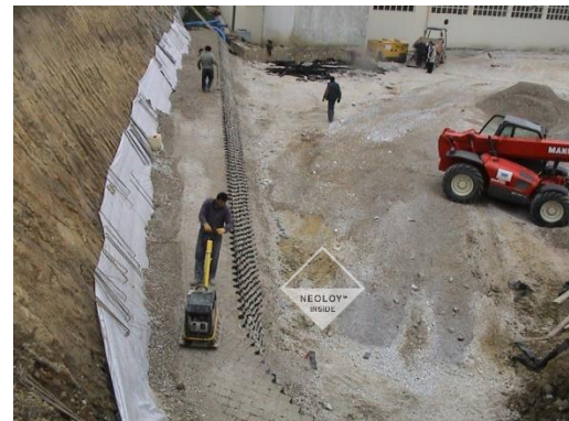
FIGURE 21. MANUAL COMPACTION WITH VIBRATORY PLATE
