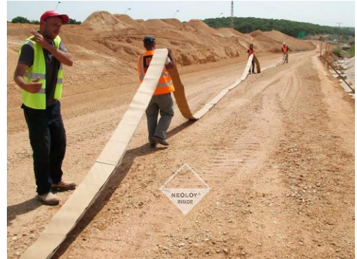
FIGURE 14. LAYOUT SECTIONS ALONG CREST OF WALL
