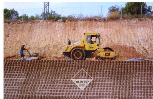
FIGURE 22. MANUAL COMPACTION OF NEOLOY ALONGSIDE MECHANICAL COMPACTION OF BACKFILL
