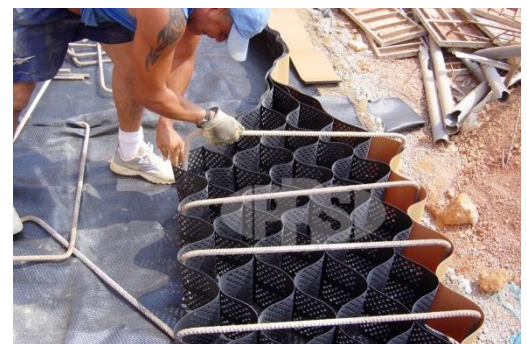
FIGURE 16. ANCHOR WITH U-SHAPED REBARS
