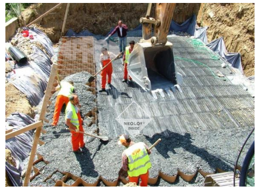
FIGURE 17. INFILL PLACEMENT
