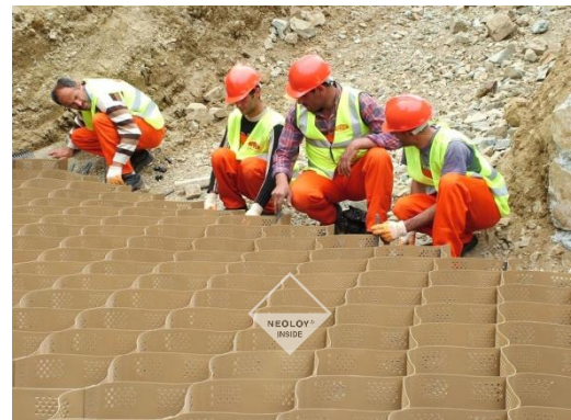
FIGURE 12. EXPANDING SECTIONS OVER ANCHORS
