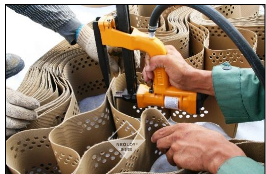
FIGURE 11. FASTENING SECTIONS FACE TO FACE
