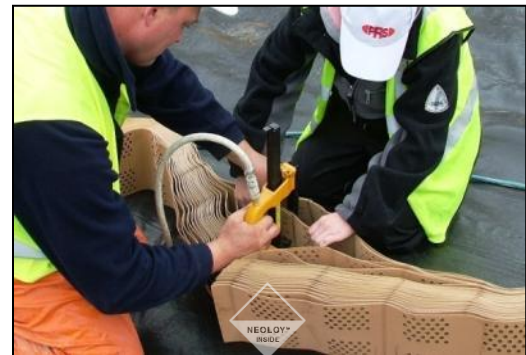
FIGURE 13. FASTENING END TO END
