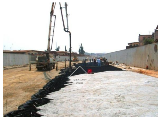
FIGURE 26. CONCRETE INFILL OF CHANNEL BED
