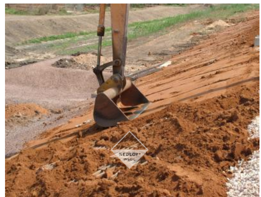
FIGURE 24. BLADE COMPACTION
