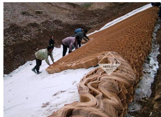
FIGURE 20. EXPANDING SECTION DOWNSLOPE
