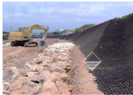
FIGURE 21. ANCHORING END OF SECTION IN TOE-TRENCH IN CHANNEL BED (INFILL WITH BOULDERS)
