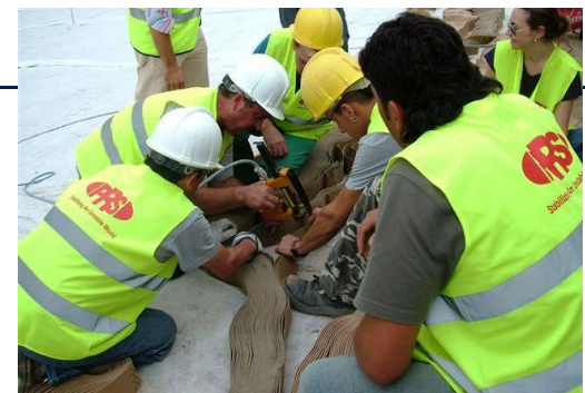
FIGURE 14. FASTENING SECTIONS FACE TO FACE
