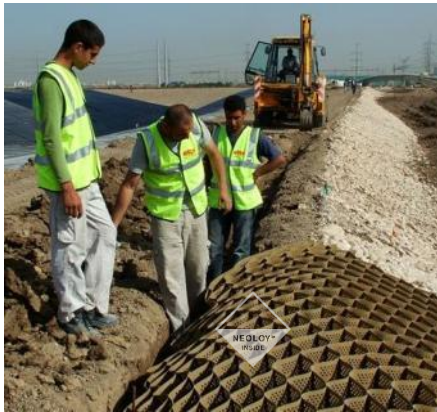
FIGURE 17. PLACING SECTION ON ANCHORS IN CREST TRENCH
