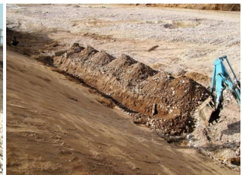
FIGURE 7. TRENCH AT TOE OF CREST TO ANCHOR BOTTOM OF SYSTEM
