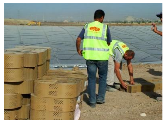
FIGURE 4. OFF-LOADING SECTIONS ON-SITE
