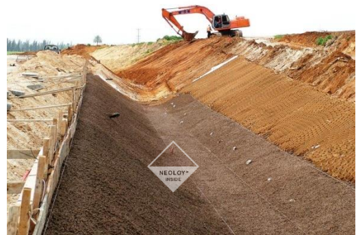
FIGURE 25. CONCRETE INFILL OF TRENCH
