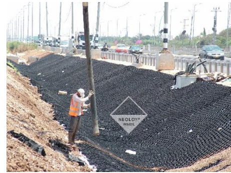
FIGURE 1. TYPICAL CHANNEL PROTECTION
