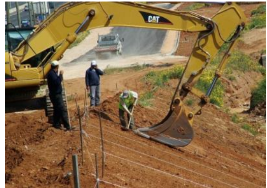
FIGURE 5. CLEAR AND SHAPE CHANNEL & SLOPES
