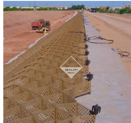
FIGURE 18. NEO-CLIPS FASTEN SECTIONS IN PLACE ON FLAT CREST SHOULDER
