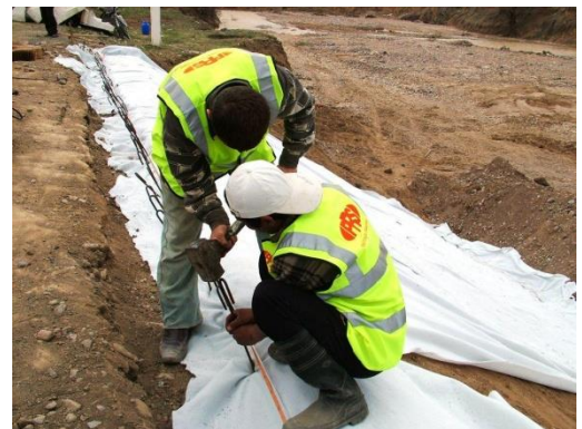
FIGURE 16. ANCHORING STAKES
