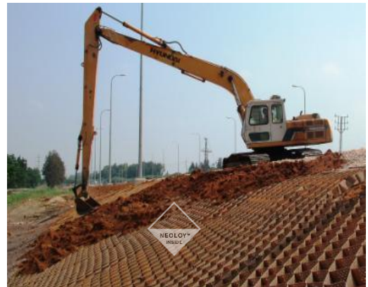
FIGURE 23. SOIL INFILL DOWNSLOPE BY EXCAVATOR
