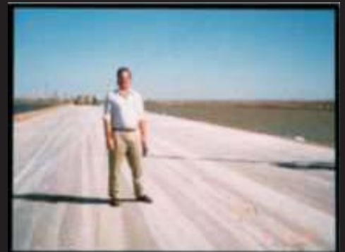
Hei Bey Road in China 1999 built over salt flats still there
